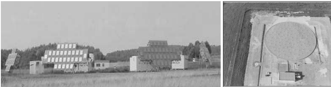
Figure 2.8: The GRAVES radar sensor. Left: transmitting antennas; right: receiving antennas (images by ONERA).
