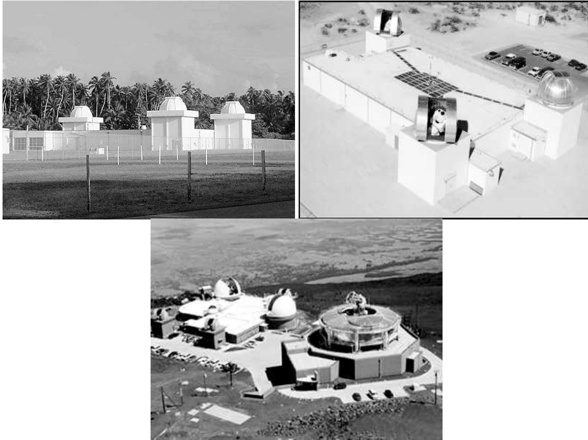
Figure 2.4: The three GEODSS sites: Diego Garcia (upper left; image courtesy of Bob Ralph and Thomas Lawson), Socorro (upper right; image by CelesTrak), and Maui (lower center; image by The Air Force Research Laboratory: Directed Energy Directorate). The lower image shows the whole Maui Space Surveillance Complex, which includes the MSSS (right building) and the GEODSS (three smaller domes on the left building).
